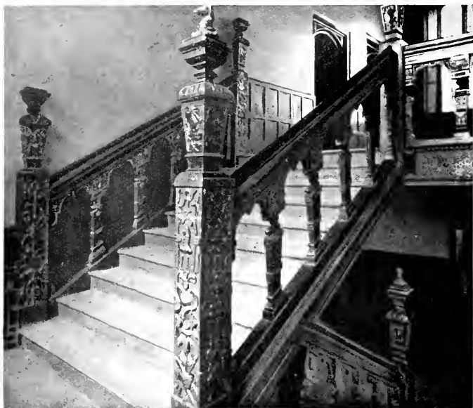
152. Staircase, The Charterhouse.
